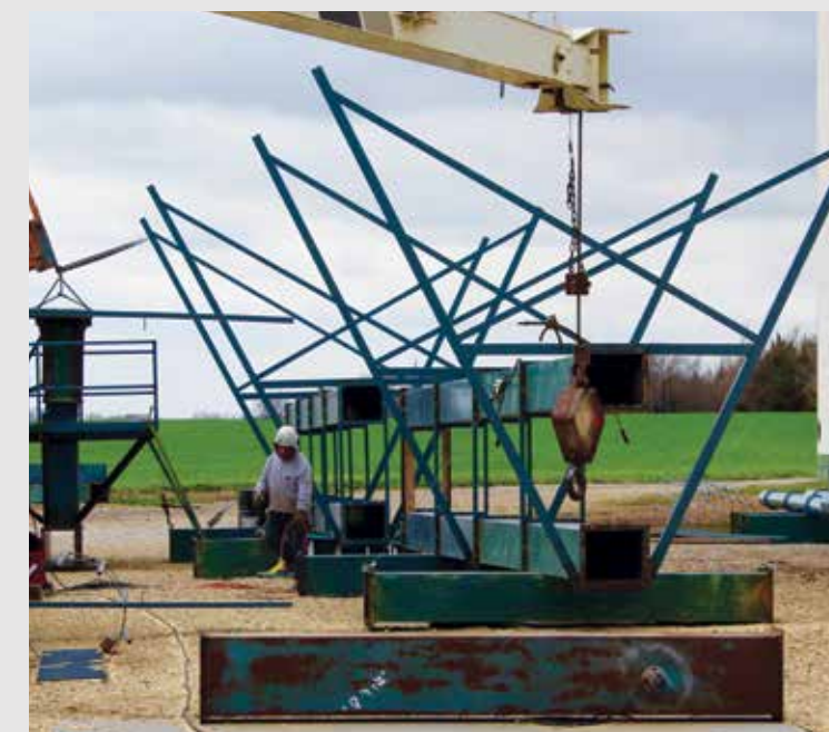
The refurbished leg will be lifted into place at Lorraine elevator.
